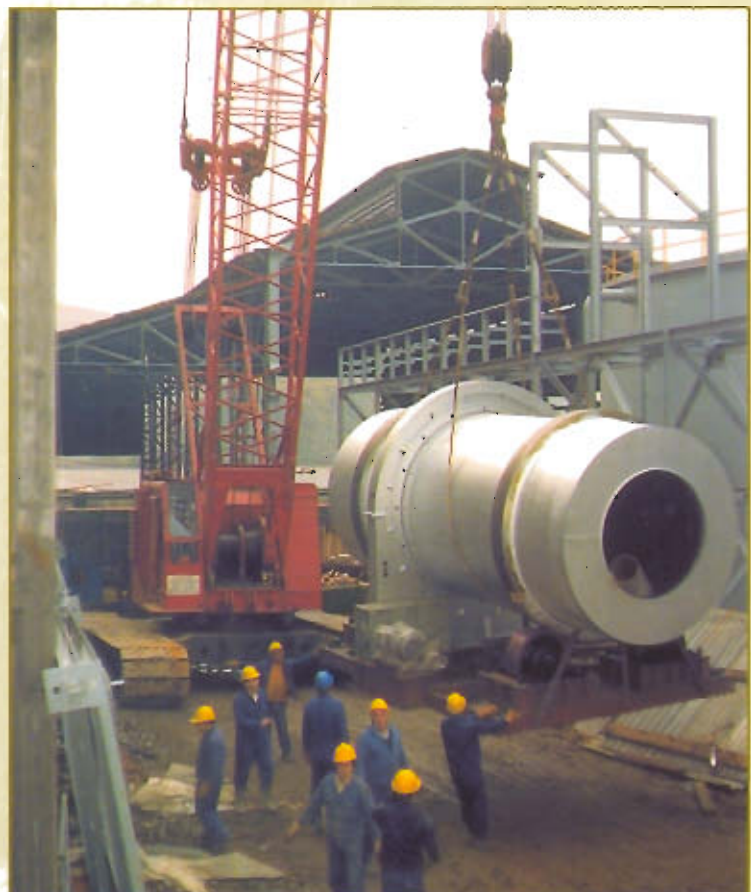
Extinguisher drum for chemical product ZAPICO-ARGENTINA
