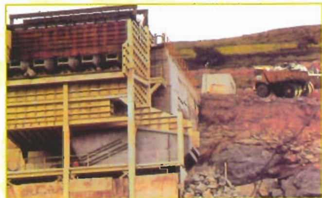
Prescreener and vibrating fingers. Classification of breakwater BILBAO -SPAIN
