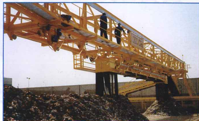
Loading framework with reversible and mobile belt: DRAGADOS TIR MADRID (Madrid, Spain) Urban Waste Materials.
