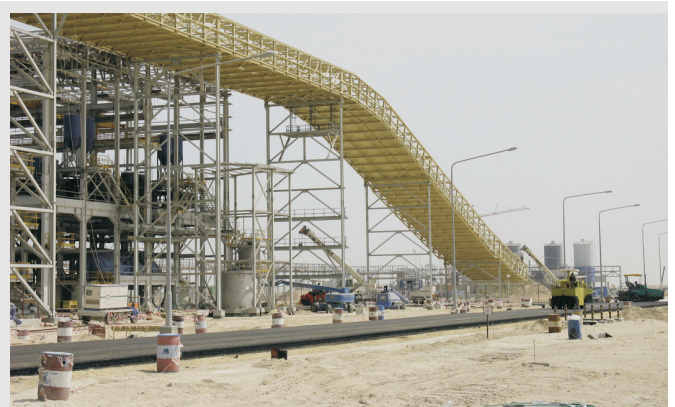
Conveyor belts (1,300 T/h), for the feeding at the MA'ADEN/WORLEY PARSONS phosphoric acid plant in Saudi Arabia. Engineering LITWIN.
