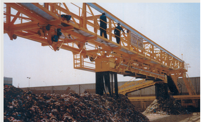
Stacker with reversible and mobile belt: DRAGADOS TIRMADRID (Madrid, Spain) Municipal Waste Materials.
