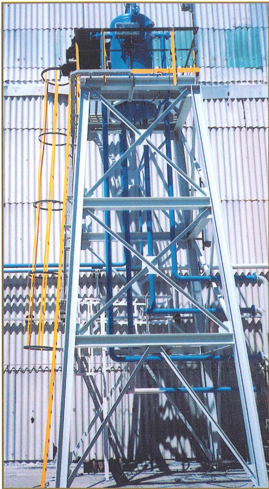
Cold air conditioning-open circuit by ammoniac evaporation.
