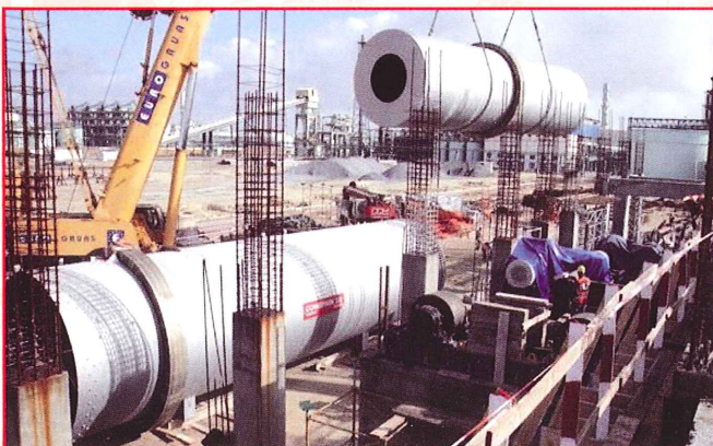
Two Dryer Drums, TSP/MAP/DAP, \varnothing 4 x 30 m, 375 T/h. BMP Bunge Maroc Phosphore (Morocco)
