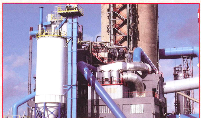
Silos and bucket elevators, Dolomite. Fertil (Annaba, Algeria).
