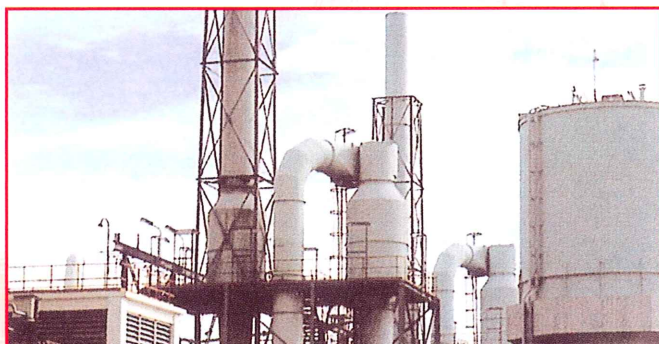
Dedusting by air-mix, 100,000 kg/h, air for ammonium sulphate dryer. E.I. Aragonesas (Huelva, Spain).
