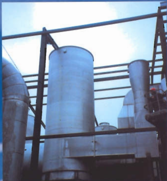
Washers with Venturi and cyclonic effect.
