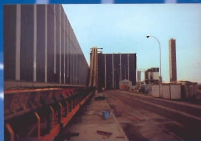
General view of feeding belt conveyors to boiler. Shown also: incinerator, system of treatment of gases and chimney stack.
