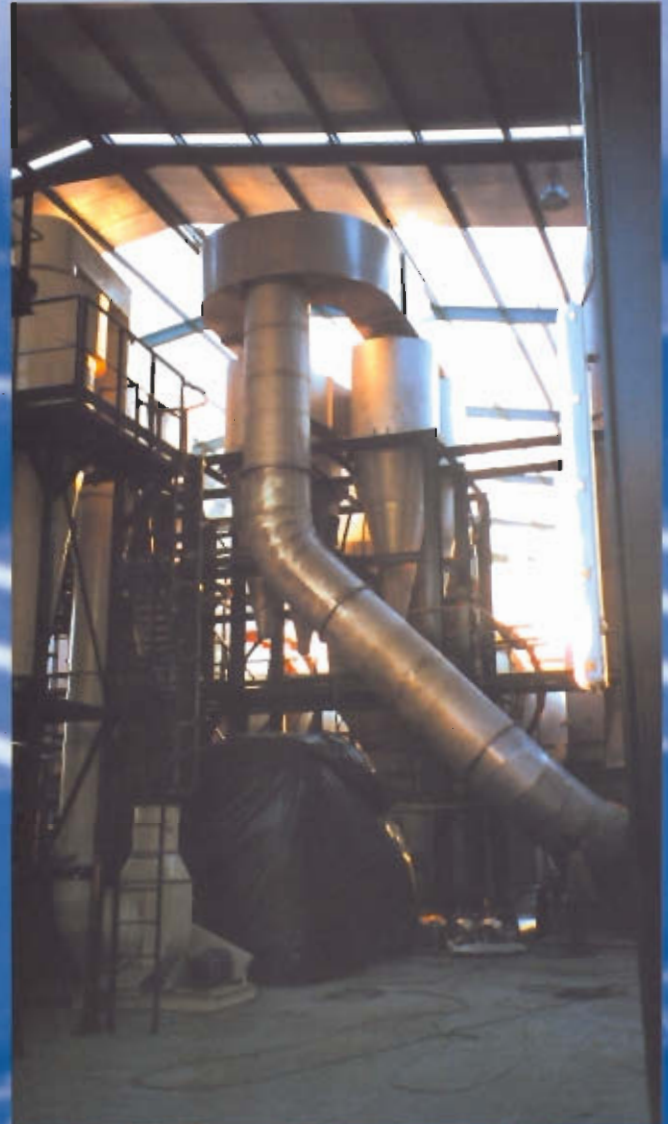
Battery of dedusting cyclones.
