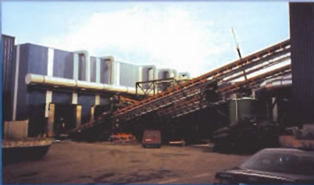
Belt conveyors of organic material to the drying area.
