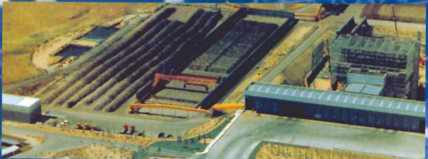
Automatically controlled fermentation park. Plant of Valdemingomez. Client: Dragados-Madrid (Spain).
