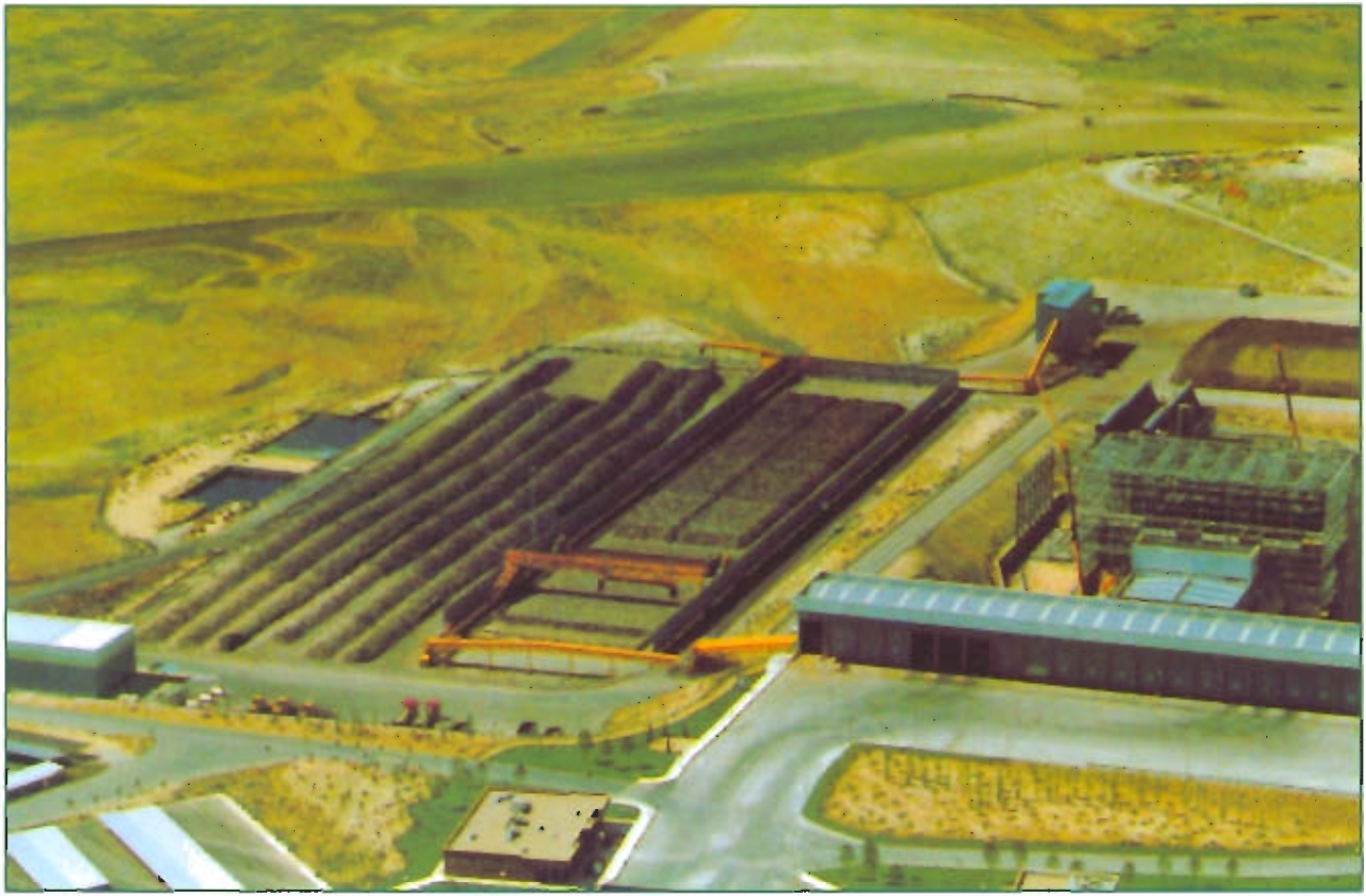
Automatic Fermentation - KOCH ESPAÑA Compost Plant Valdemingómez Plant, Customer: Dragados Madrid, (SPAIN)
