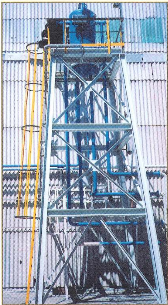
Cold air conditioning-open circuit by ammoniac evaporation.
