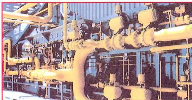
2 hot gas generators, 2 x 30,000 Th/h for TSP, PK. NPK dryers. Asmidal Annaba (Algeria).
