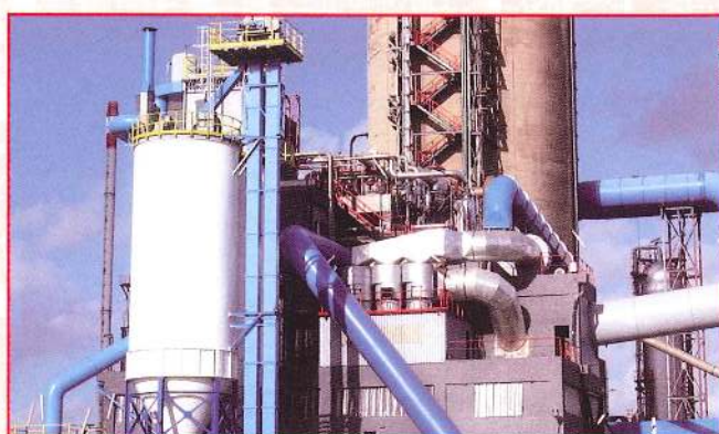
Silos and bucket elevators, Dolomite. Fertial (Annaba, Algeria).
