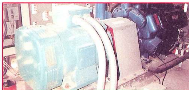
Compressor for an air conditioning unit in freon circuit, 600,000 frig/h. National Fertilizer Company – NPK plant. (Taiwan).
